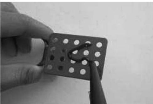
4. Orient the clip as needed on the roof. Place the roof clip on the roof where the roof is marked. Press down on the clip so that the adhesive flows through the holes. The cable insertion clamp should be vertical on the roof.
