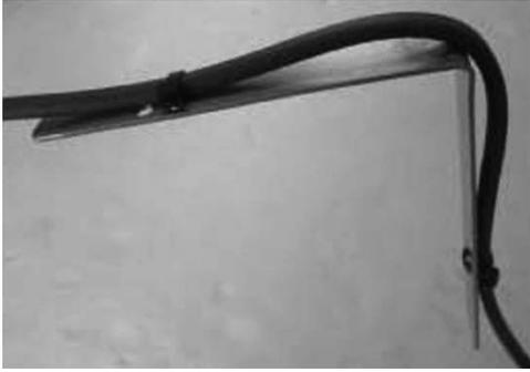
3. Make a "U" in the cable so the cable goes down the downspout and comes back up to complete the run along the remainder of the gutter.
