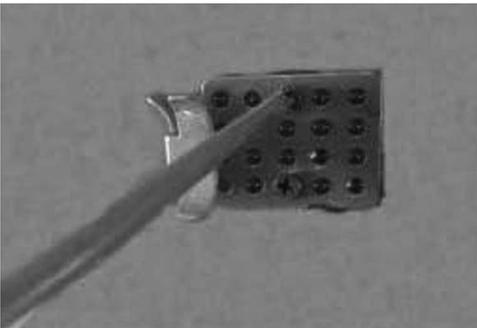
4. Apply the sealant on top of the nail or screw heads.
