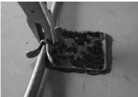
6. Run the cable from the starting point and use a roof clip to connect the cable to the edge of the roof.
