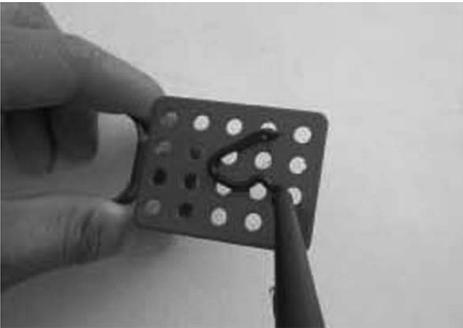
3. Orient the clip as needed on the roof. Place the roof clip on the roof where the roof is marked. Press down on the clip so that the adhesive flows through the holes. The cable insertion clamp should be vertical on the roof. Attach the clip to the roof using a nail or a screw.
