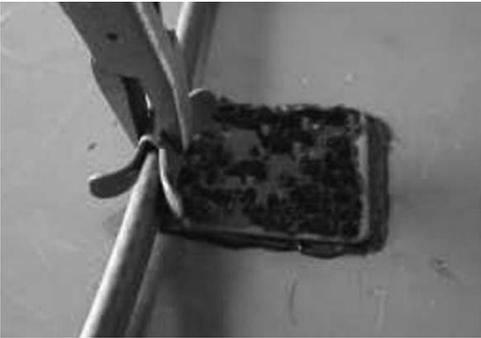
8. Run the cable from the starting point and use a roof clip to connect the cable to the edge of the roof.
