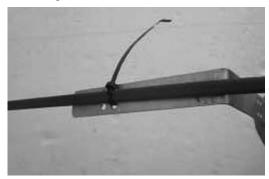
2. Tighten the cable ties to secure the cable. Trim off the excess ends of the ties. Do NOT cut the heating cable.
